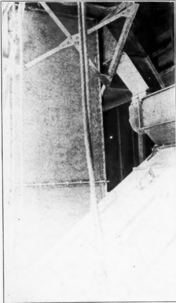
Elevator and Chute to Vibrating Screen
